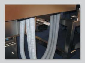
Classification according NEN-EN-IEC 61386: Compression resistance: Class 4, Heavy (1250 N). Impact resistance: Class 4, Heavy (6 J). Tensile strength: Class 4, Heavy (1000 N). Protection class: IP 67 (dust-proof, water-tight).
